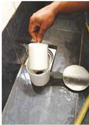
3 Remove the bell cap (by lifting it from the container).
