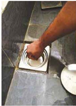
2 Remove the water seal trap (container & bell cap).
